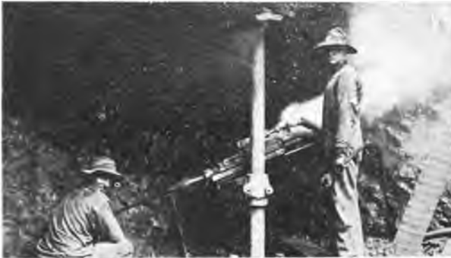
B. DRILLING BY STEAM IN ST. LOUIS LODE, 1911.
